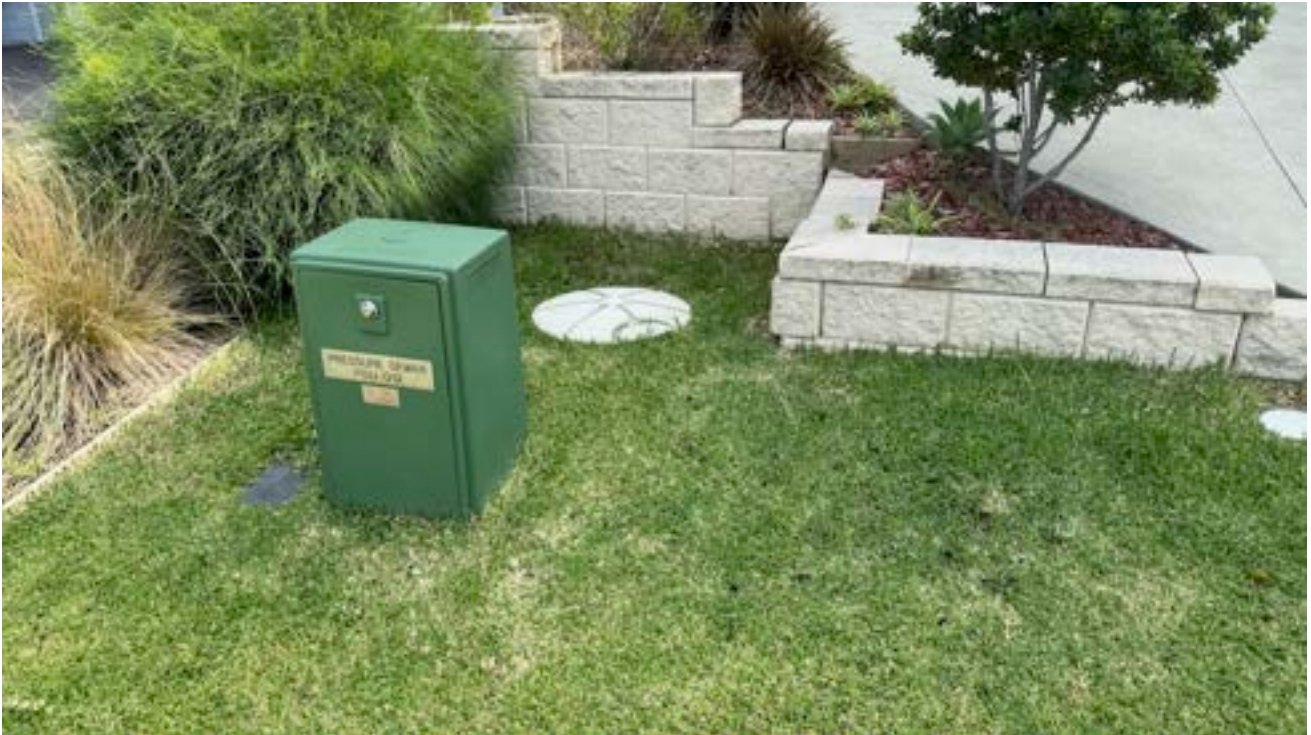
Figure 7. Established sewer connection (Anouska Street) showing intact and accessible structures.
