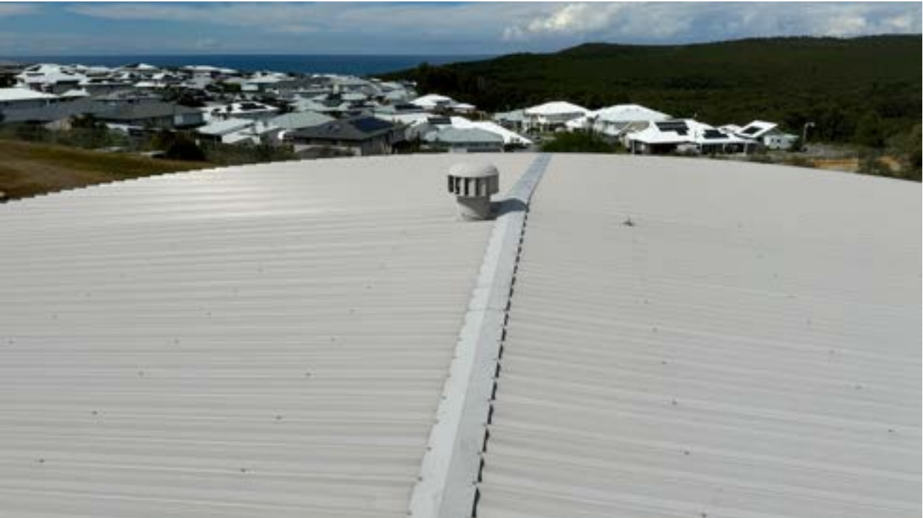
Figure 1. Overview of closed water storage tanks inspected, showing them to be ostensibly in good condition.
