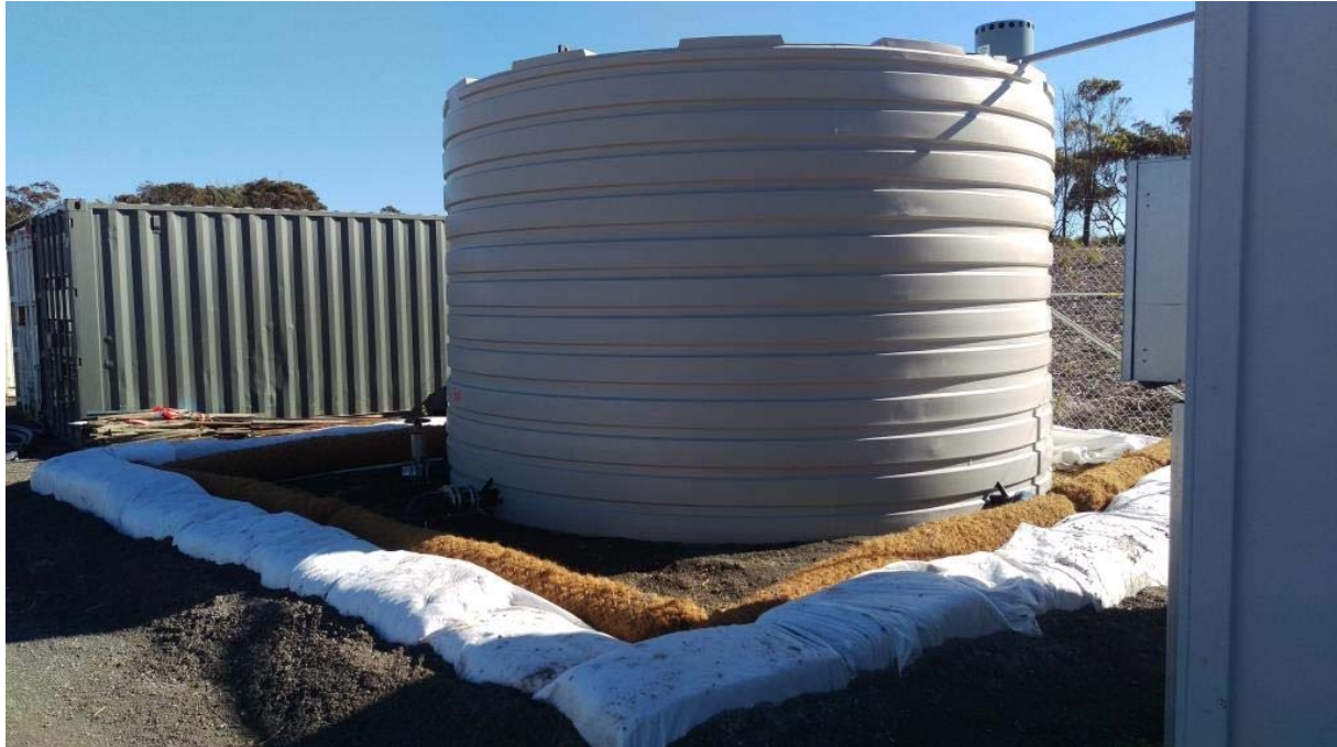
Figure A.5.1 Sewage Pump Out Tank showing (a) carbon filter fitted at the top of the tanks; and (b) bunding immediately around the tank.
