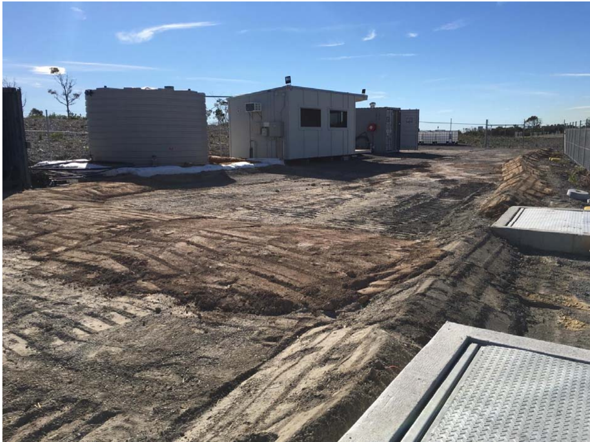
Figure A.5.9 Earth bunding around perimeter of site is in place to capture sewage spills. Note that bunding immediately around the Sewage Pump Out Tank remains in place.
