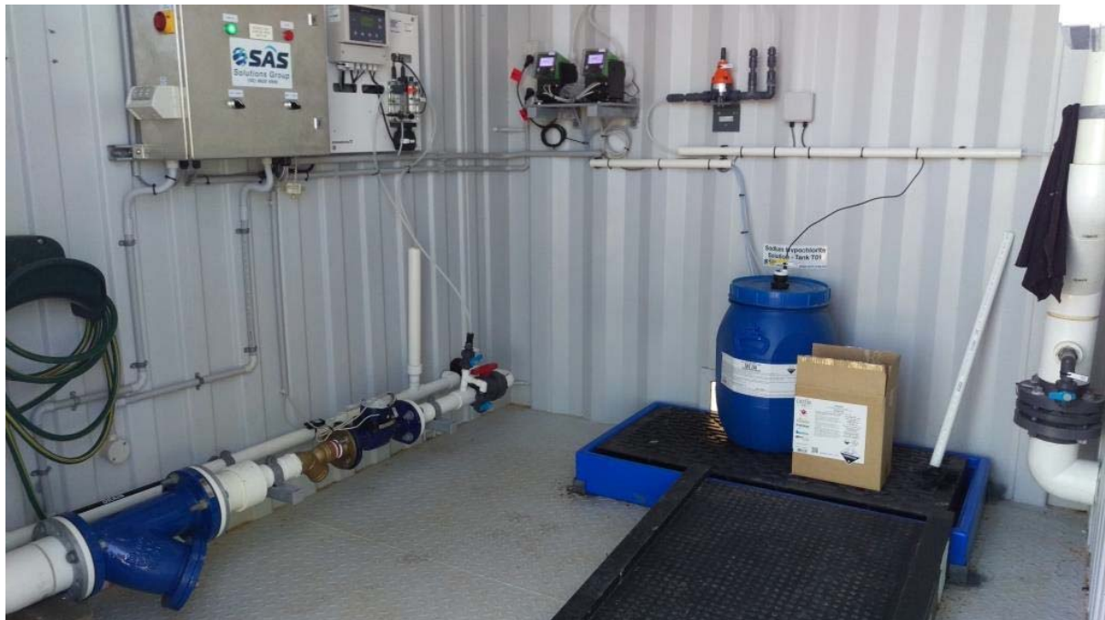
Figure A.5.8 Chlorinator Room.
