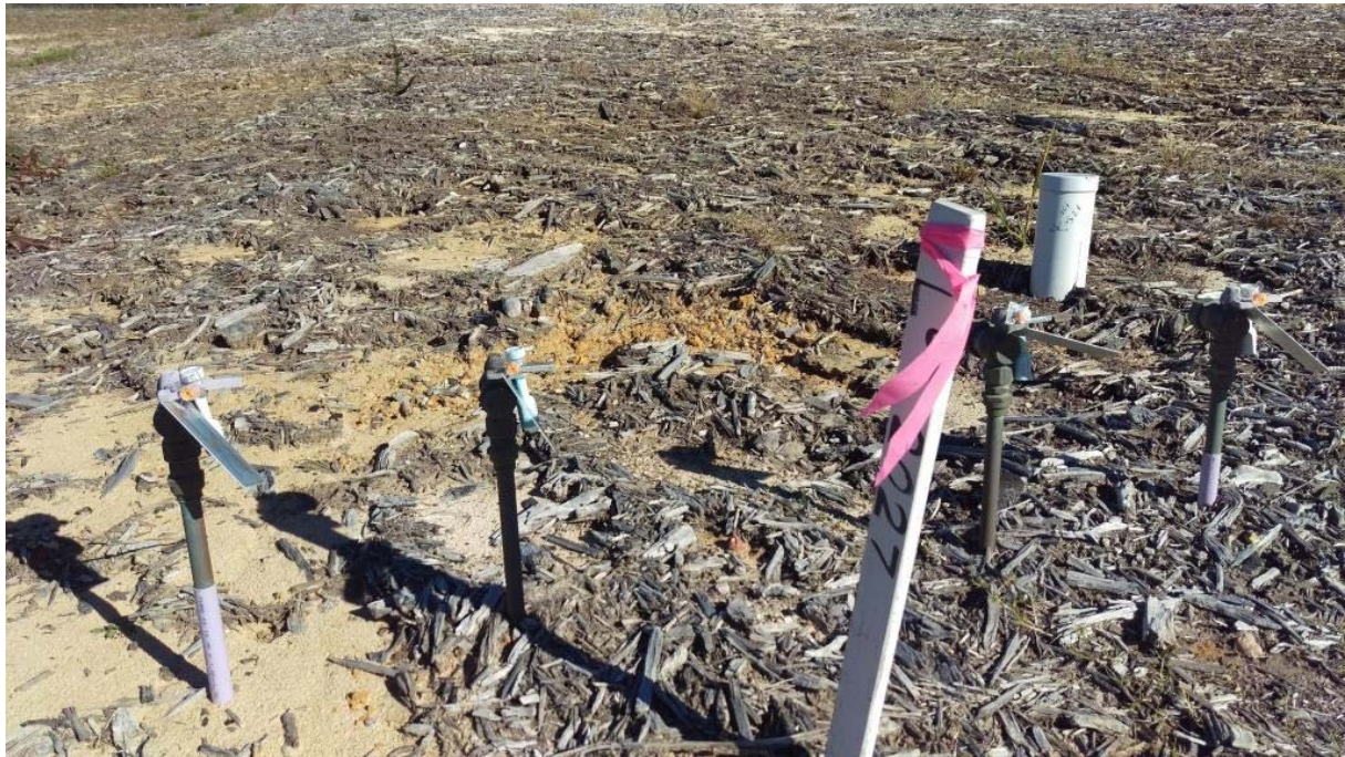
Figure A.5.5 Property service connections showing (a) lilac sleeving and isolation valve on recycled water connection; and (b) appropriate separation between drinking water and recycled water services.
