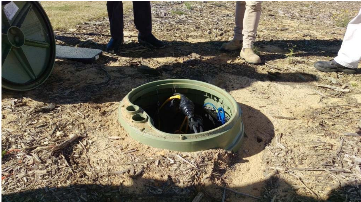
Figure A.5.2 Pressure Sewer Unit showing (a) discharge pipework from submersible pumpsets; and (b) cover with rubber seal (at left).
