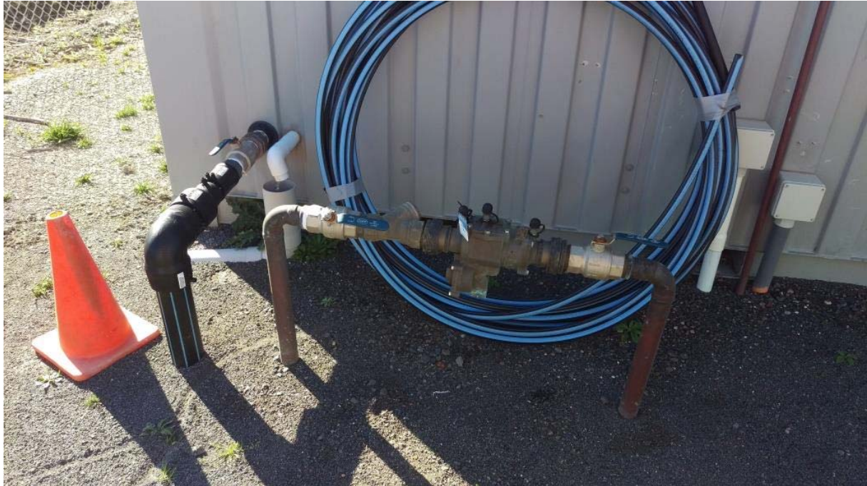
Figure A.5.7 Backflow prevention on domestic supply to the site office (and ultimately the treatment plant site). Test tag is in place.
