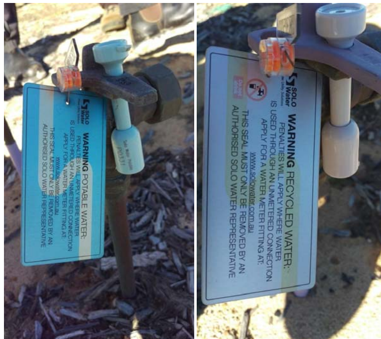
Figure A.5.6 Property service connections are appropriately sealed and tagged.
